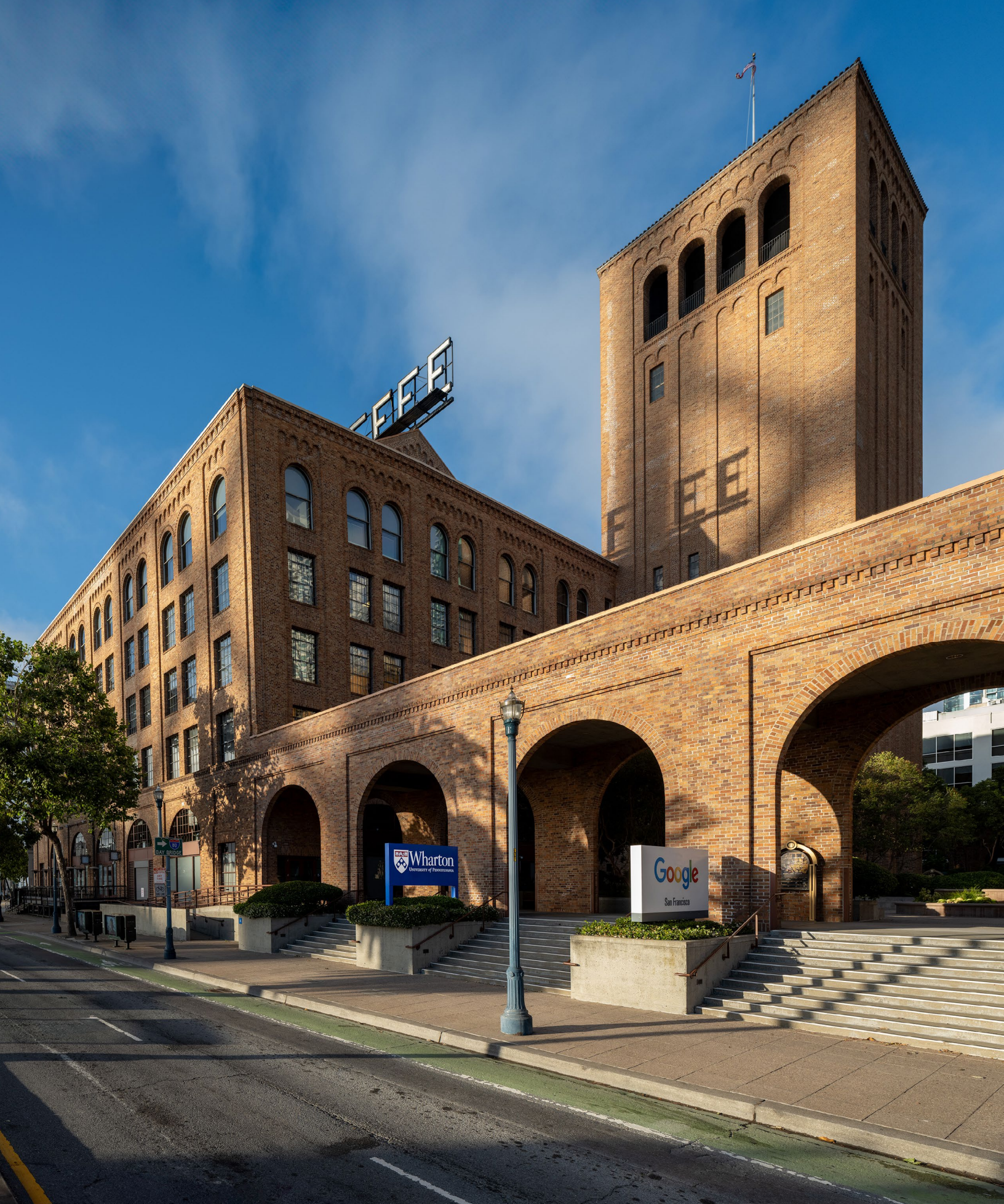
The Hills Brothers Coffee Building in San Francisco, CA
